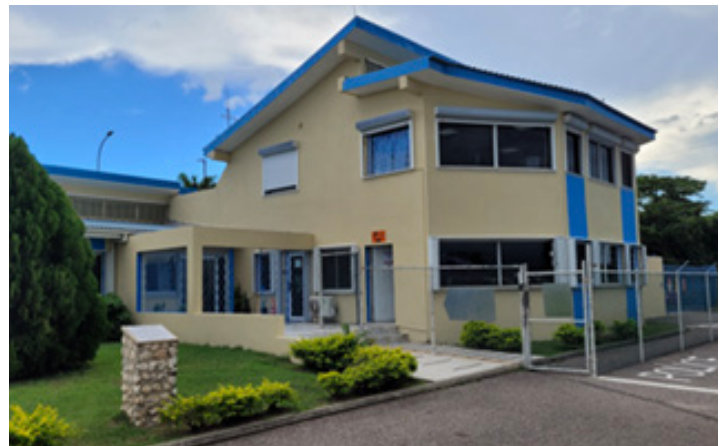
Repainting exterior of Vineyards Toll Plaza
