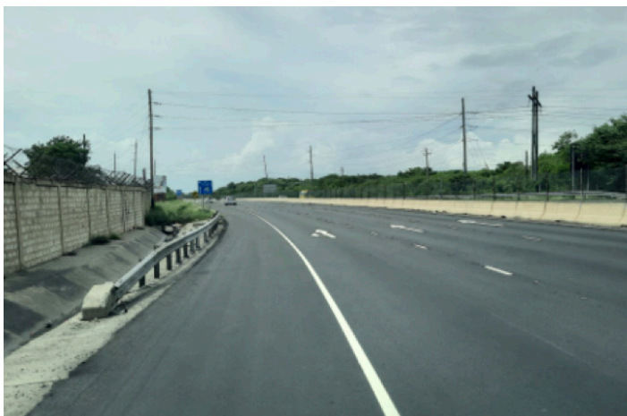
Asphalt overlay Marcus Garvey Interchange westbound with new lane markers installed.
